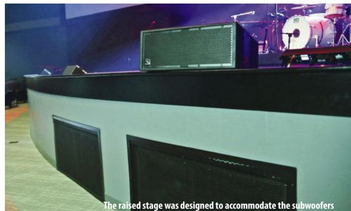
The raised stage was designed to accommodate the subwoofers
